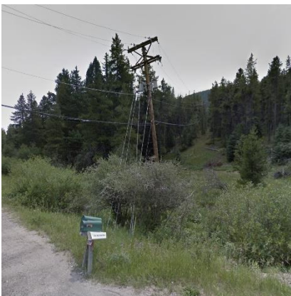
Existing Shadow Mountain Drive Overhead Powerline Corridor
